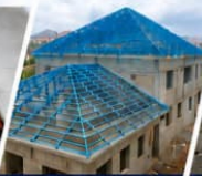
STEEL TRUSS & ROOF STRUCTURE
