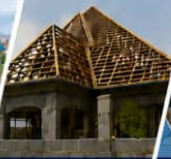
ROOF CONSTRUCTION & INSTALLATION
